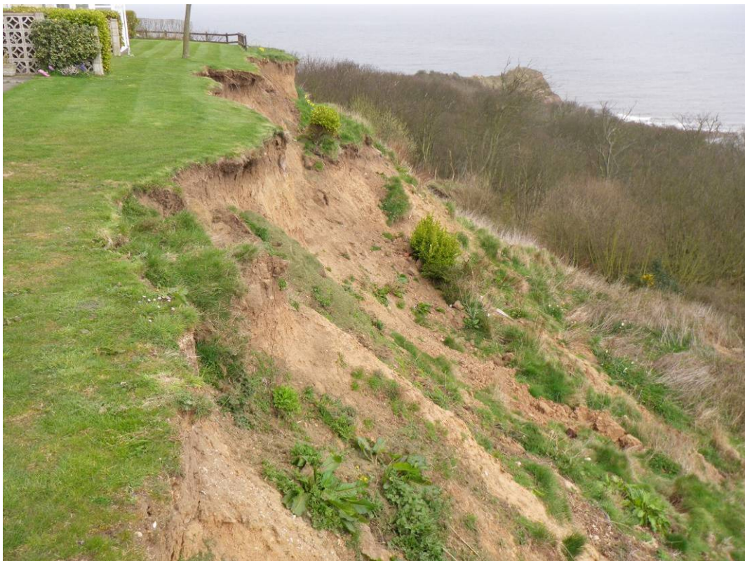
Plate 14 Cliff recession at Knipe Point Headscarp looking east (14 th April 2010)
