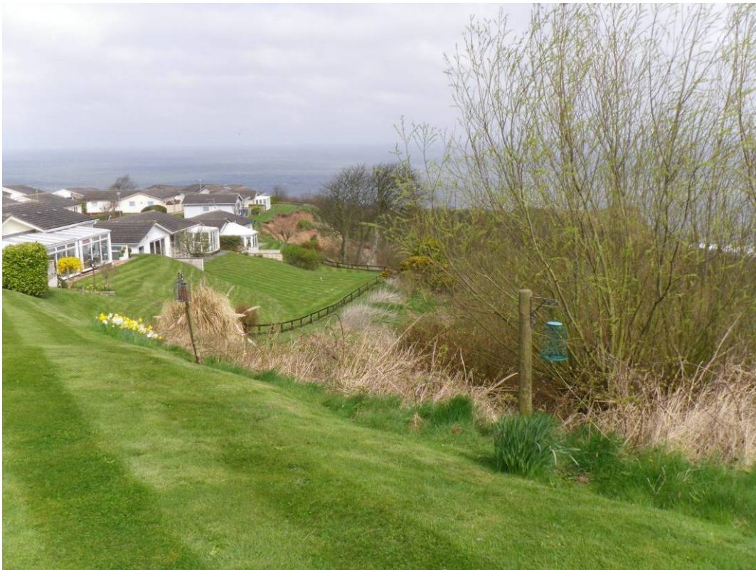
Plate 16 Cliff recession at Knipe Point Headscarp looking east (14 th April 2010)
