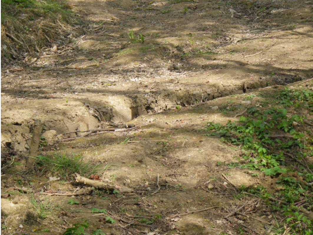
Plate 2 Tension cracks trending northeast / southwest landward of BH05
