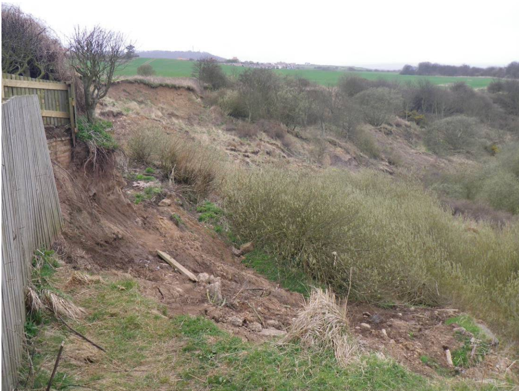
Plate 3 Slope failures on Cornelian Bay side of Knipe Point looking northwest
