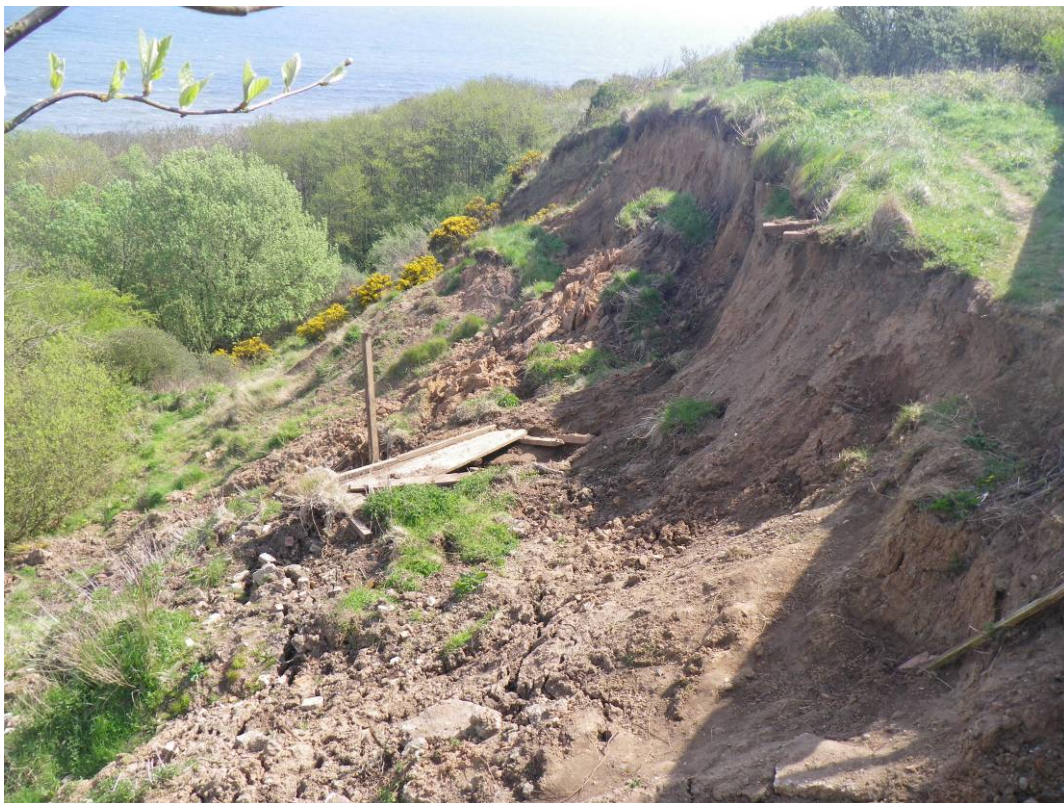
Plate 6 Slope failures on Cornelian Bay side looking east (5 th May 2010)
