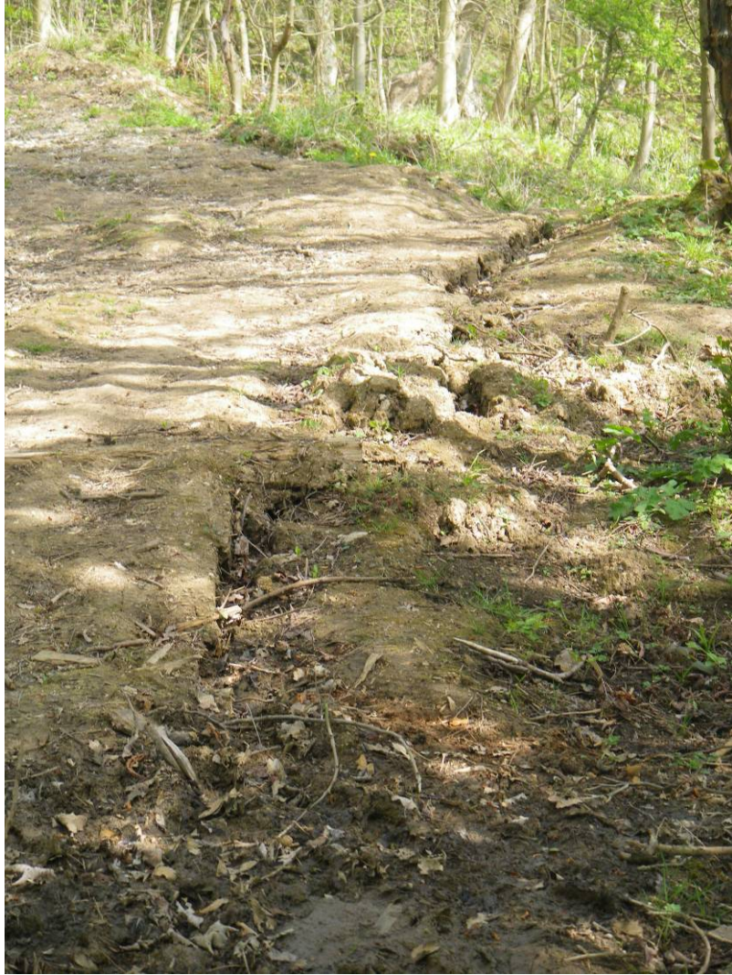
Plate 1 Tension cracks trending northeast / southwest landward of BH05
