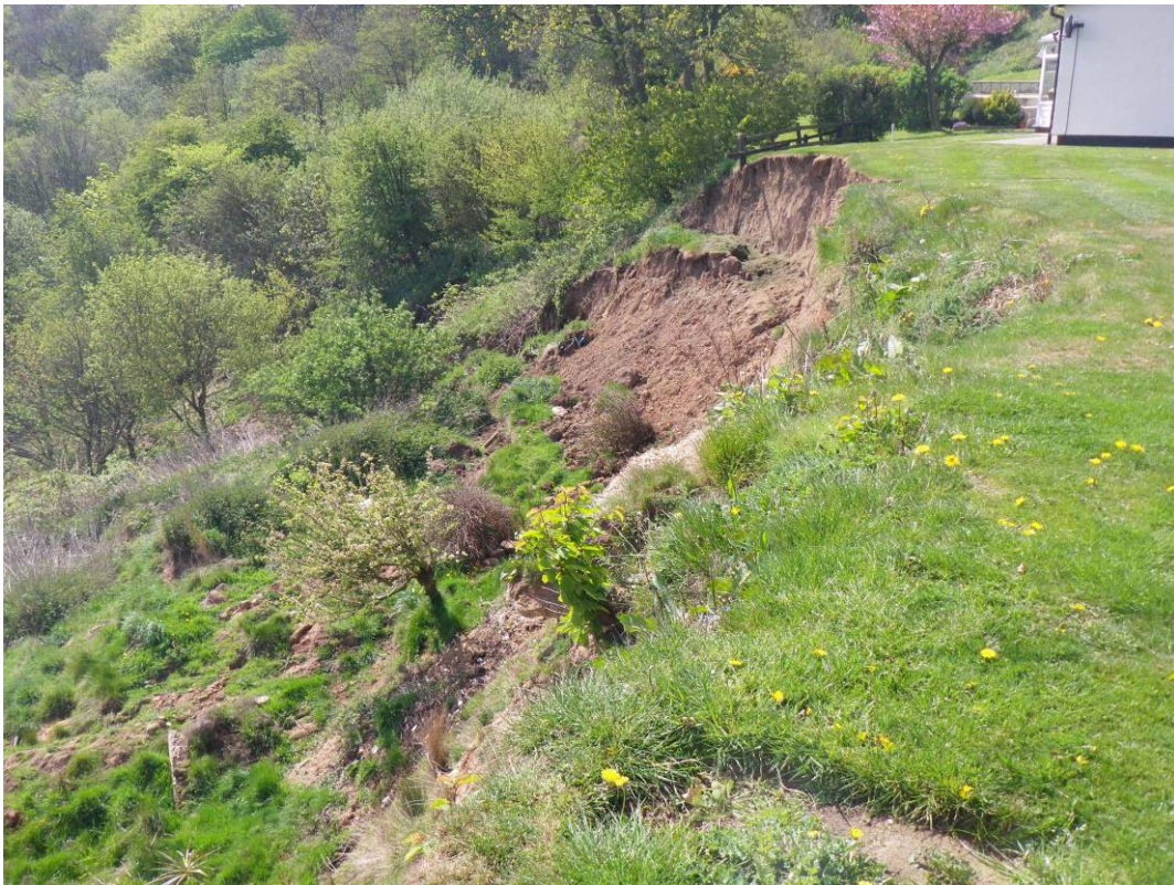
Plate 12 Cliff recession at Knipe Point Headscarp (5 th May 2010)
